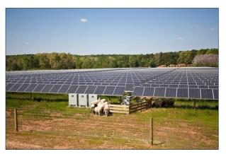
The electricity is cabled to inverters, which convert DC power to AC, synchronised to the electricity grid. The output is connected through various switchgear, protection devices and meters to local users and the grid.
