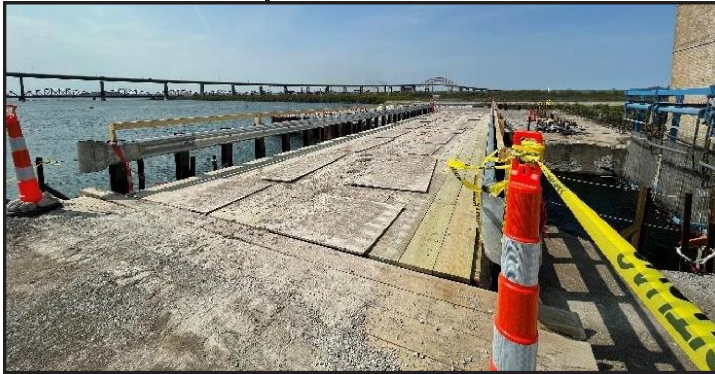
Prefabricated steel bridge installed west of Unit 10, providing haul route access to the Center Dike fill area
