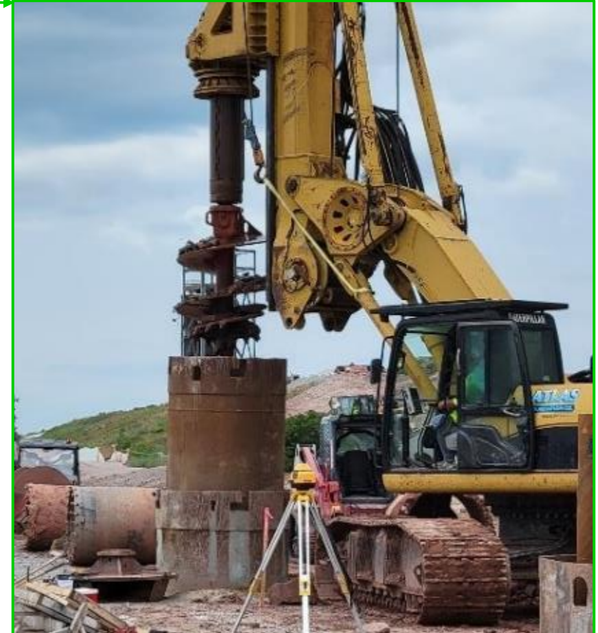
Drilled shaft installation of concrete panel deadmen
