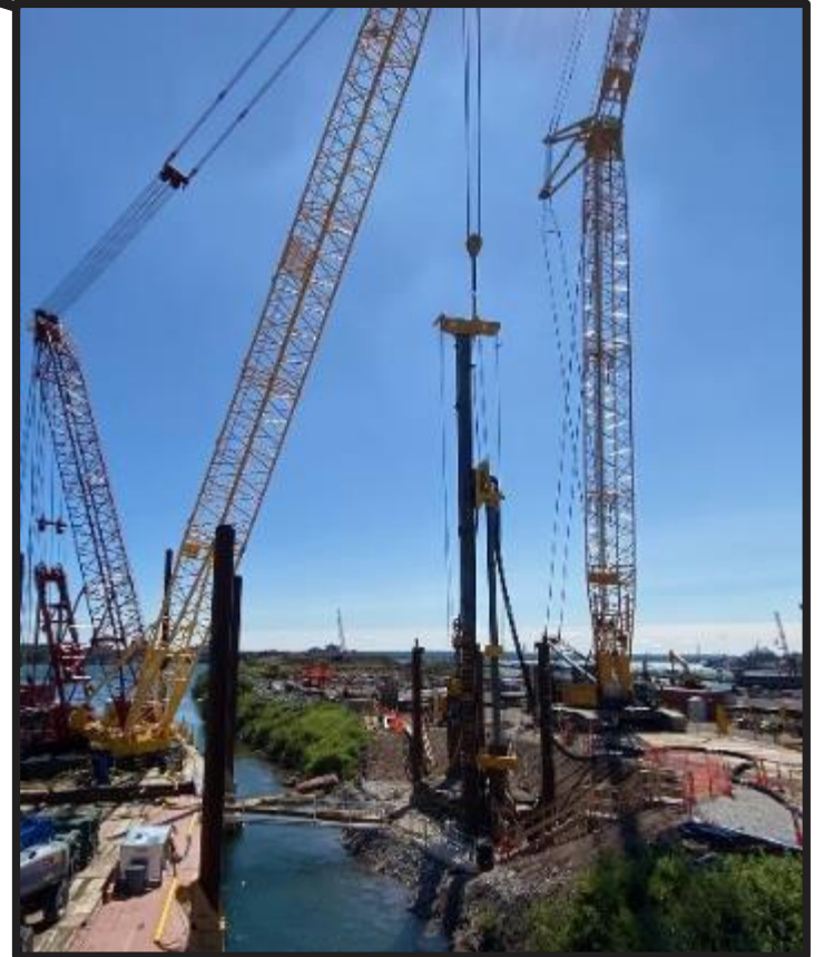
Drilled shafts for NPP Bridge south pier abutments
