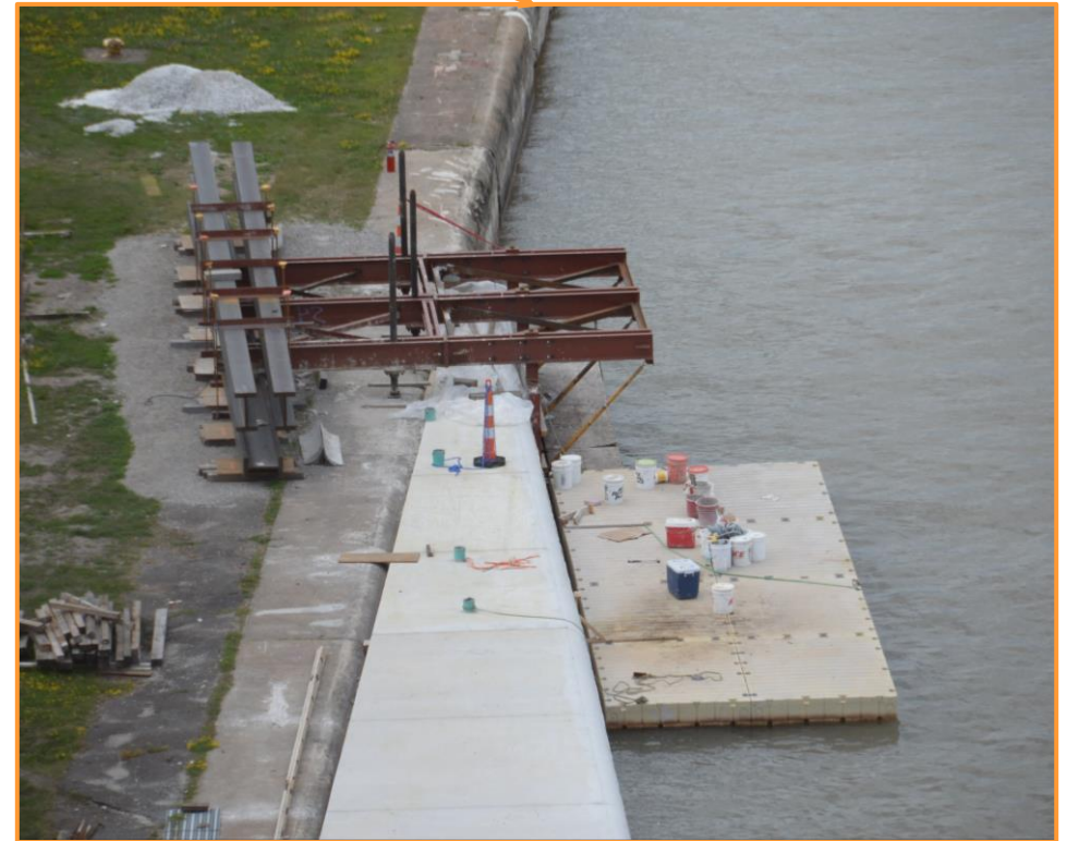
Southwest SSP transition wall with concrete cap
