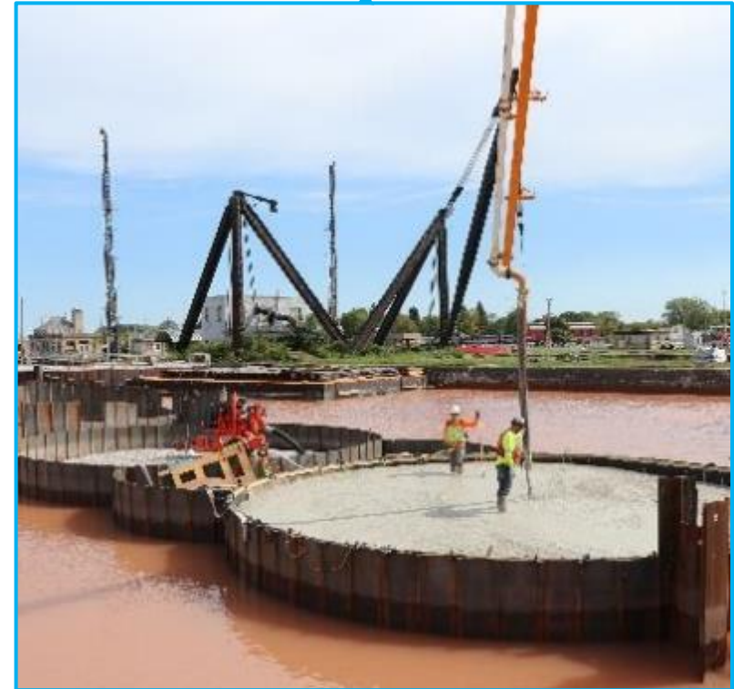
Concrete placement in cell
