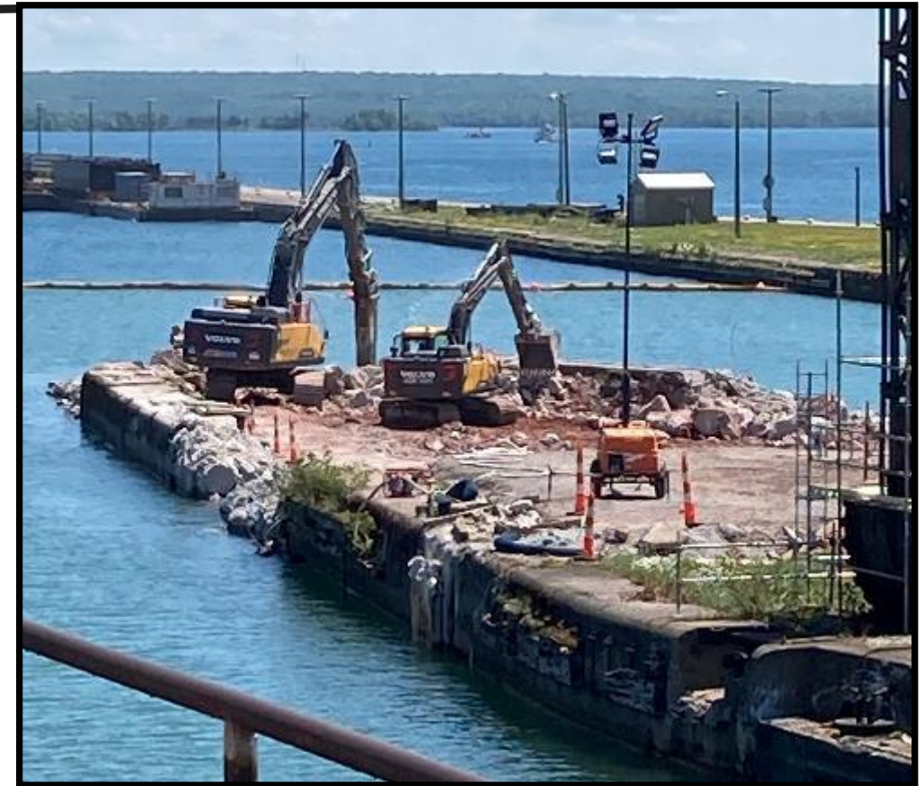
Demo of Downstream Nose Pier in preparation for downstream cofferdam construction
