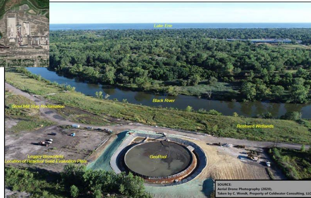
Top photo: BRDMRF location along south side of Black River. Bottom photo: BRDMRF Dewatering GeoPool Pilot Study (Source: Coldwater Consulting, LLC, 2020).
