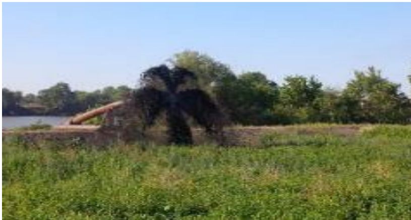
Dredged Material being pumped into Facility
