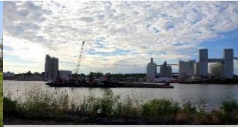
Barge of Dredged Material Transported to Facility
