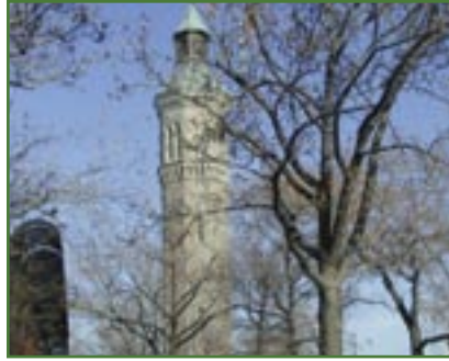
Highbridge Water Tower
