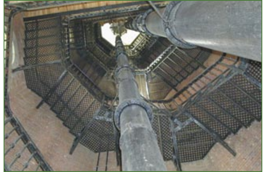
Highbridge Water Tower Interior
