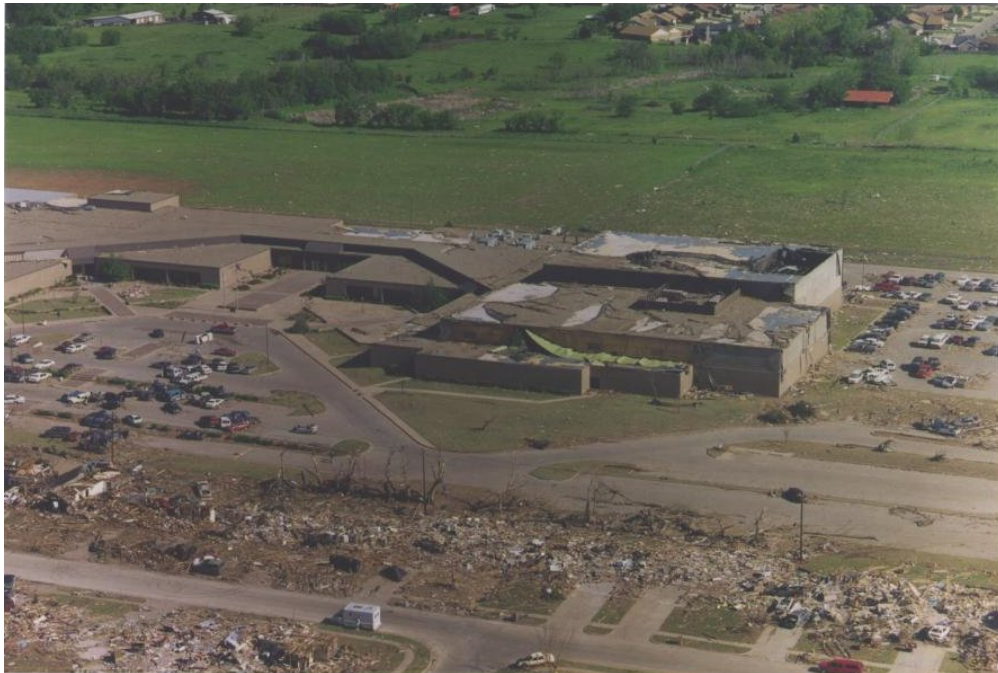
ES: DOD 5: Significant loss of roofing material (>20%); uplift of roof decking
