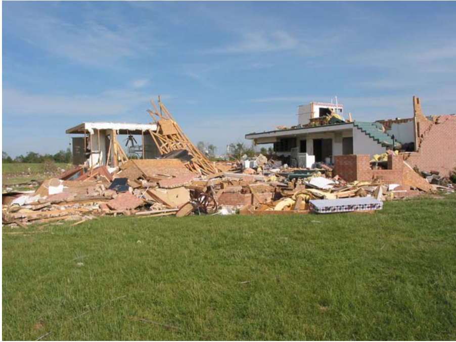
FR12: DOD 10: Total destruction of entire building
