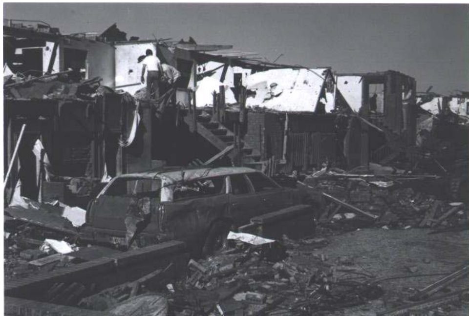
ACT: DOD 5: Most top story walls collapsed
