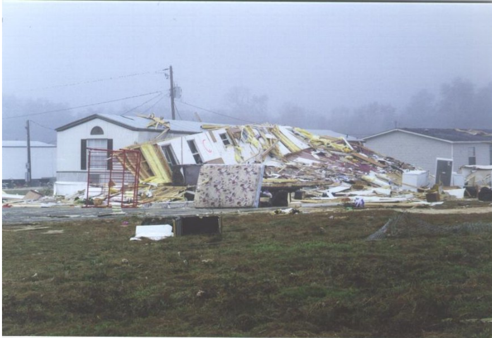
MHSW: DOD 6: Destruction of roof and walls leaving floor and undercarriage in place
