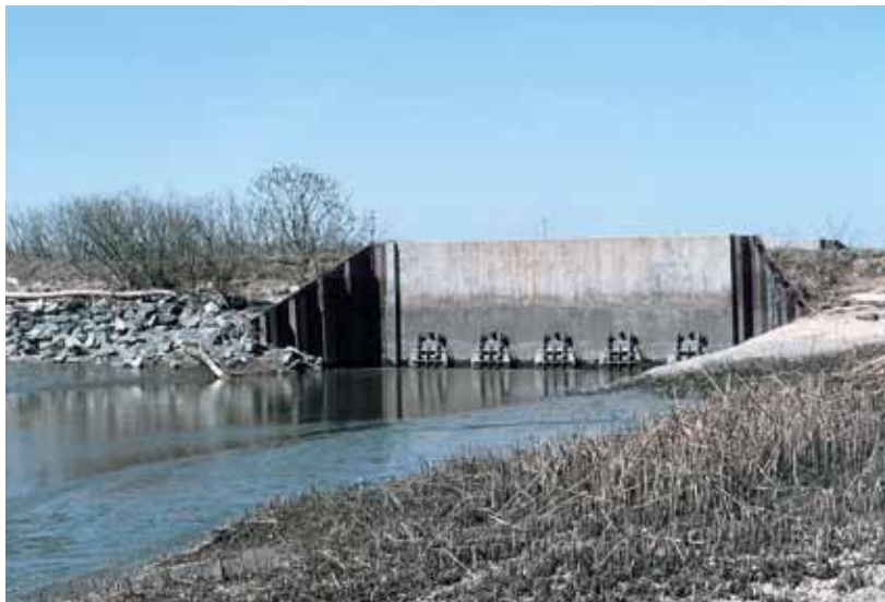
NOAA Restoration Center
