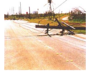
Weakened, unguied wooden power poles can break
