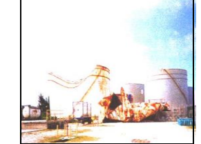
Tops of empty fuel storage tanks can be stripped away
