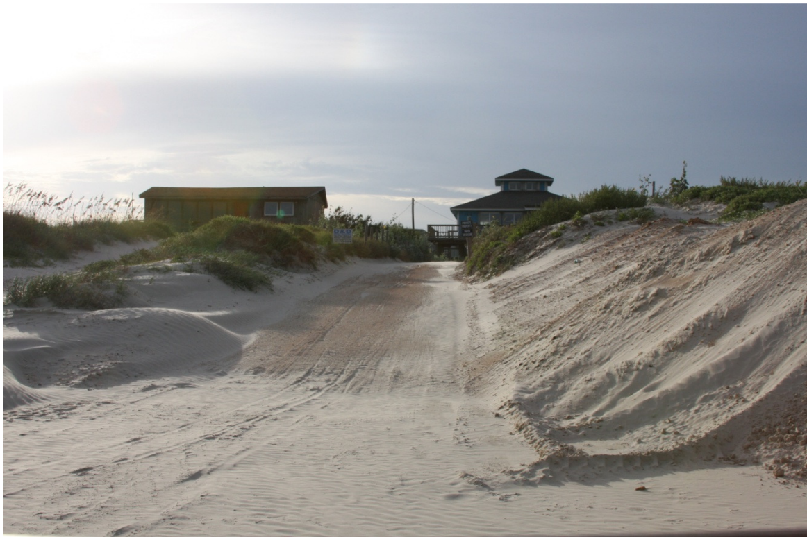
Figure 4. Dunes with a typical driveway breach and home behind
