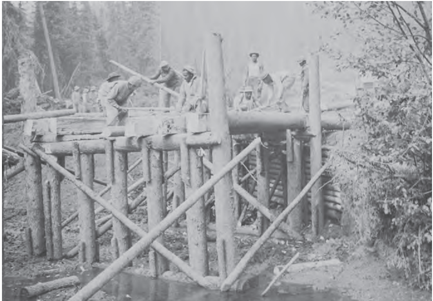
Soldiers of the African American Ninety-Fifth General Services Regiment at the Sikanni Chief River Bridge, British Columbia, 1942. NWCS/H Reed, National Archives and Records Administration, College Park, MD. Photo No. 111-SC-139940.
