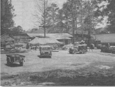
The remains of Camp Castle in June 1989. (U.S. Army photo by Pvt. Bryant Griffin)
