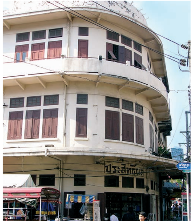
House in Wang Li community
