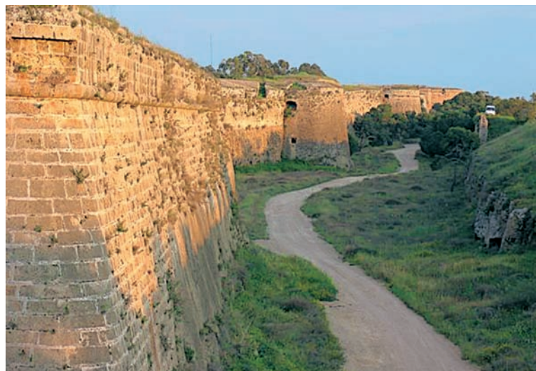
Fig. 6 The fortified walls and moat of Famagusta
