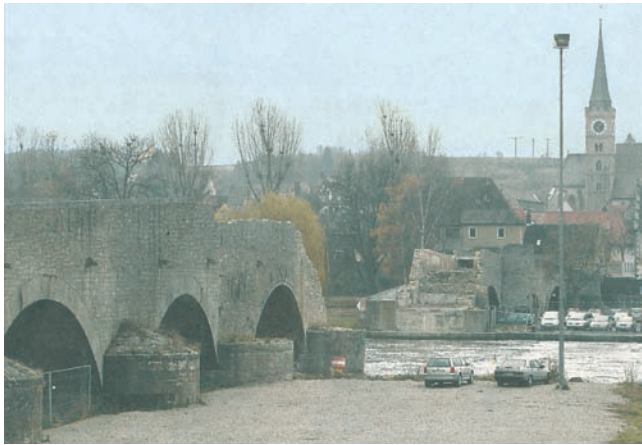
Ochsenfurt, old bridge across the river Main (Photo: Weissbach)
