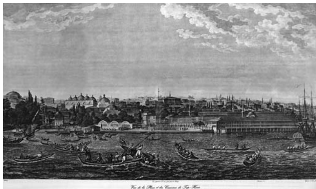
Fig. 15 Tophane (Melling’s Panorama 21, 1819). This panorama presents the Tophane place situated on the European shore of the Bosphorus with vast barracks and other representative still existing buildings: the Kılıç Ali Paşa Mosque built by architect Sinan, the Tophane fountain(1732) and the gunfoundry vaulted with six domes. It forms a highly representative urban prospect and scenery of the distinguished residential Pera quarter including the harbour with splendid ships in the foreground
