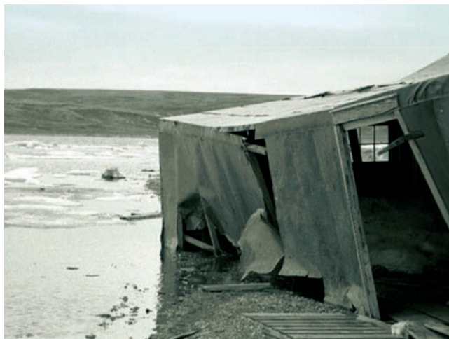
June, 2001 - the NW&TCo Store shed addition after being crushed by sea ice the previous fall (Credit: Government of Yukon Territory)
