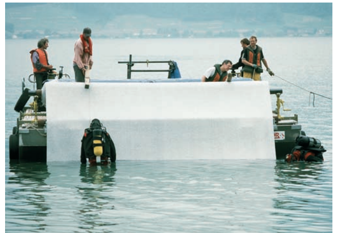
Erosion protection measures at Lake Biene, Switzerland (2003-2004). 'ROBOR' catamaran in action with geotextile mats. 6,000 m2 of the settlement site in the bay of Sutz-Lattrigen have been covered over and 30,000 m2 have been excavated archaeologically. Photograph: Archaeological Service Canton Berne.
