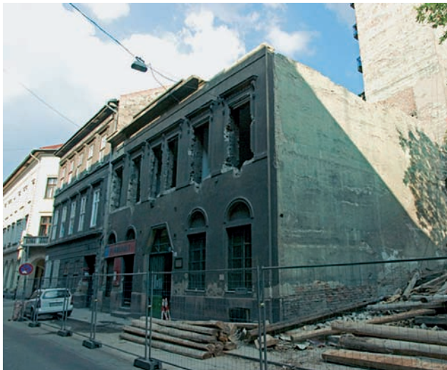
Demolition of Dob Street
