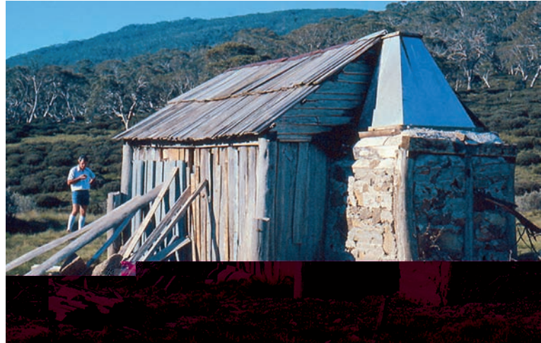
Burrungabugge Hut, which was destroyed by the 2003 bush fires and not reconstructed. This hut itself replaced another hut burnt down in 1983.
