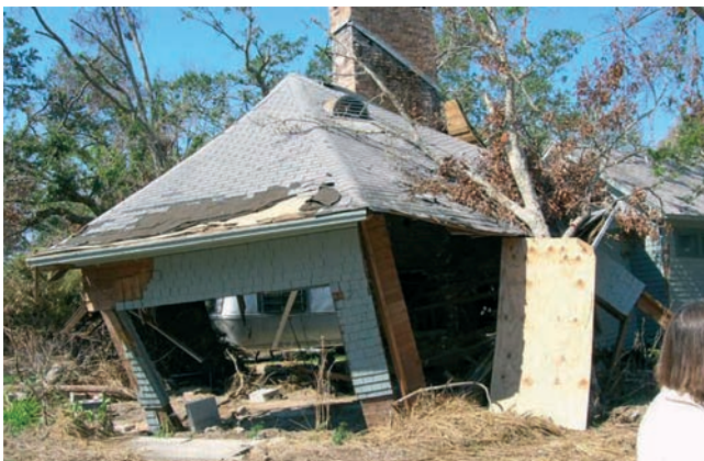
Badly damaged house designed by Frank Lloyd Wright
