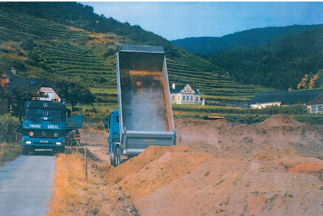
Duernstein, construction work in front of the Kellerschloessel
