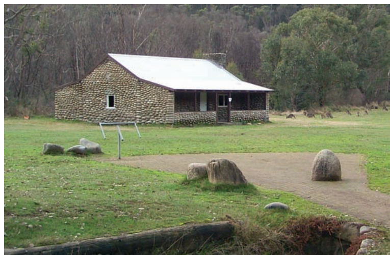
Geehi Hut, burnt out in the 2003 bush fires and in part restored and in part reconstructed in 2004
