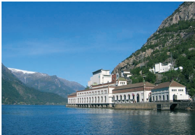
The Tyso hydropower plant (1906-16) is today a national monument and beautifully restored after its closure in 1996 (Photo: Axel Mykleby)
