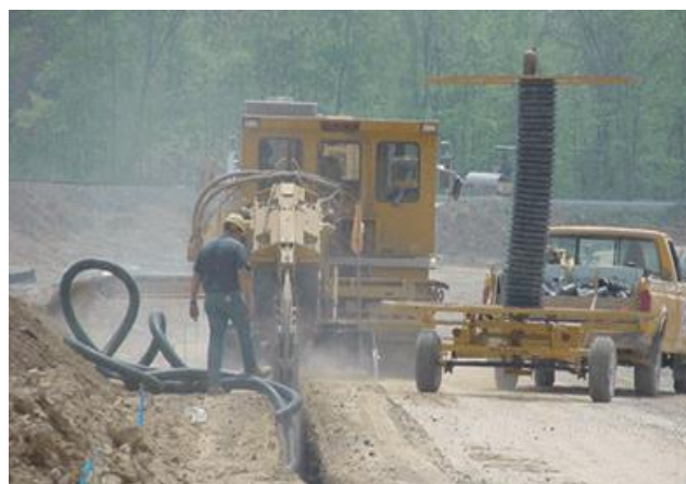
FIGURE 27: UNDERDRAIN INSTALLATION.
