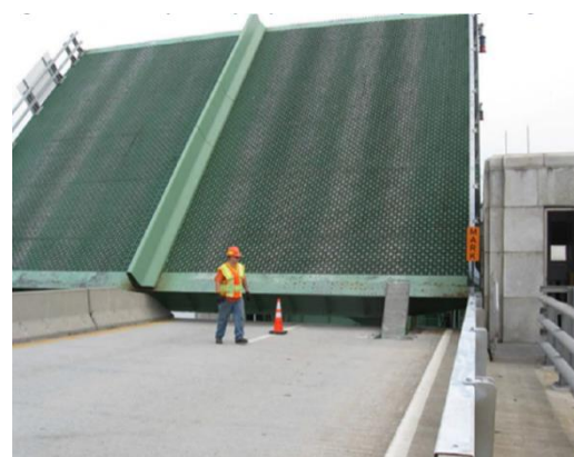
FIGURE 30: THE BASCULE BRIDGE ON LOOP PARKWAY OVER LONG CREEK.
