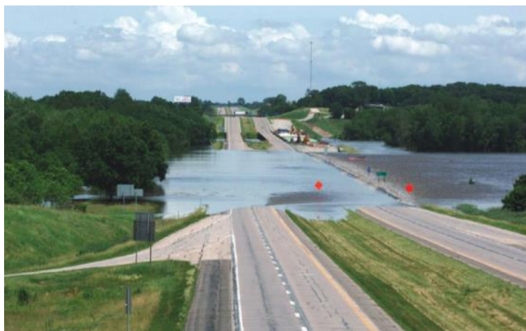
FIGURE 19: FLOODING OF I-80 NEAR CEDAR RAPIDS, IOWA. Source: IDOT Pilot study.
