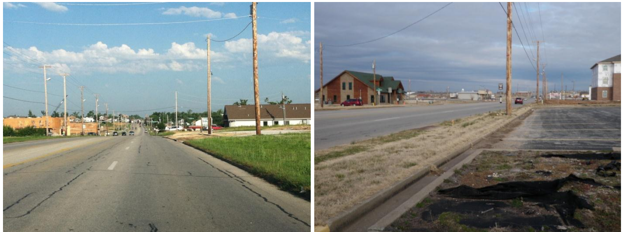
Figure 7: Both images show the lack of sidewalks on either side of the roadway, which discourages pedestrian use of the corridor.
