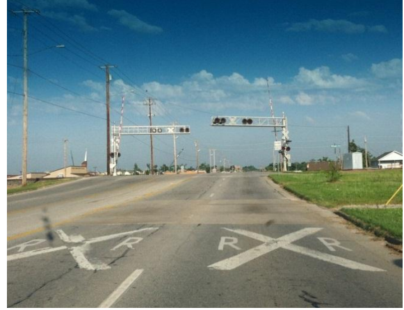
Figure 19: East 20th Street looking west at the future viaduct location.
