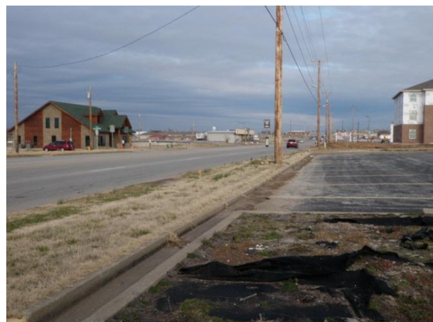
Figure 14: Minimal available ROW outside of the roadway in this location near South New Hampshire Avenue.
