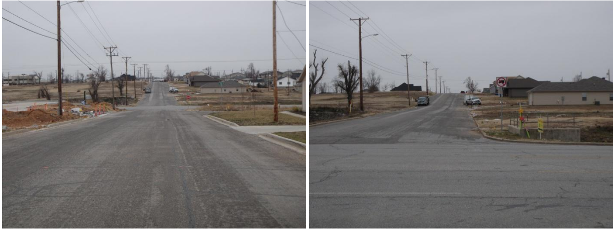
Figure 8: Images of South Highview Avenue showing the wide pavement width.
