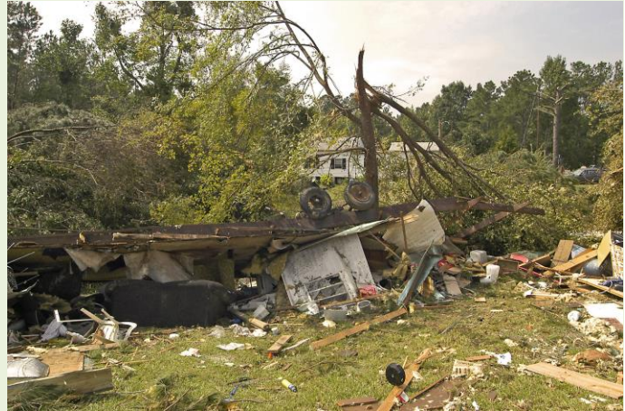
Figure 2. Tornado damage at a mobile home park in Ridgeway, South Carolina (FEMA).
