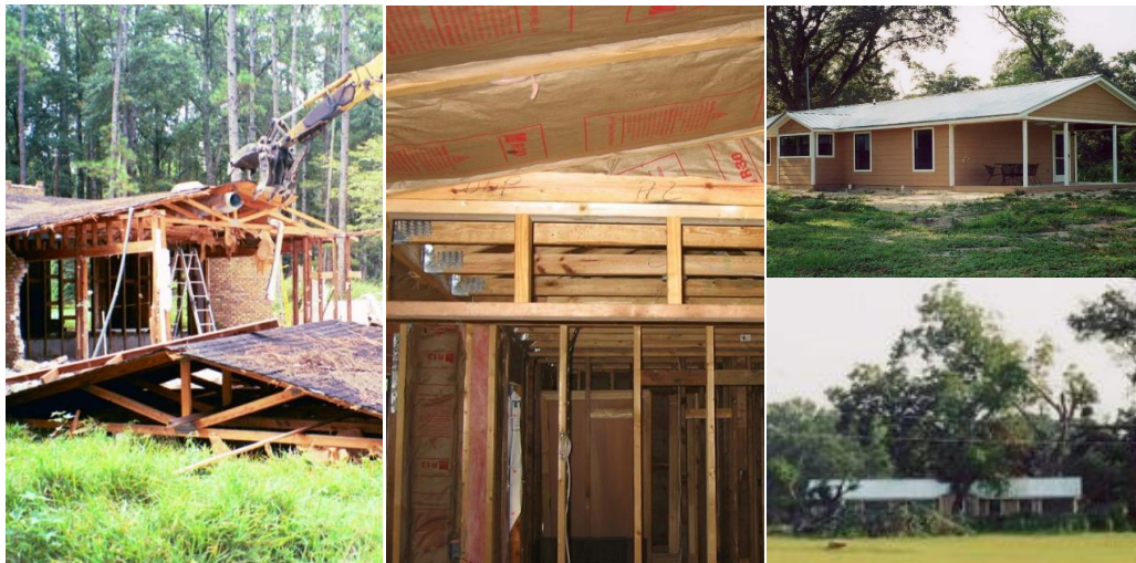
Figure 23. Panelized deconstruction was used to deconstruct a home in a floodplain buyout in Alachua County, Florida, and the lumber was used to build new Section 8 affordable housing inland (Brad Guy).
