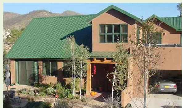
Figure 18. Top: Ceramic tile roofing is a best practice to mitigate embers from igniting the roof structure. This home was protected by its ceramic roof during the Valley Fire in Middletown, California (Adam Dubrowa / FEMA). Middle: FEMA graphic on the importance of clearing gutters (FEMA). Bottom: Home in New Mexico that incorporates fire safety measures, such as metal roofs and exterior doors, adobe and stucco exteriors, and defensible space (FEMA).
