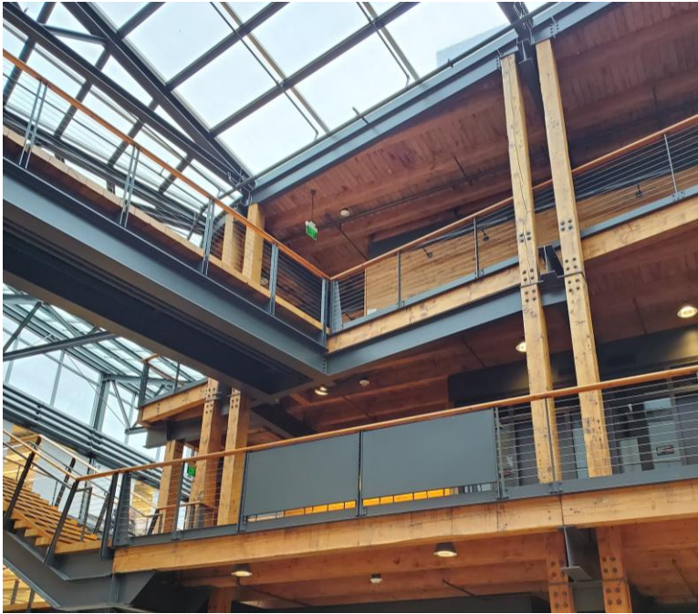
Figure 24. The Federal Center South U.S. Army Corps of Engineers Seattle District Headquarters building is a LEED Gold building completed by GSA in 2012, using nearly 200,000 board feet of structural and nonstructural lumber from an adjacent warehouse that was deconstructed (Theresa Blaine, EPA).
