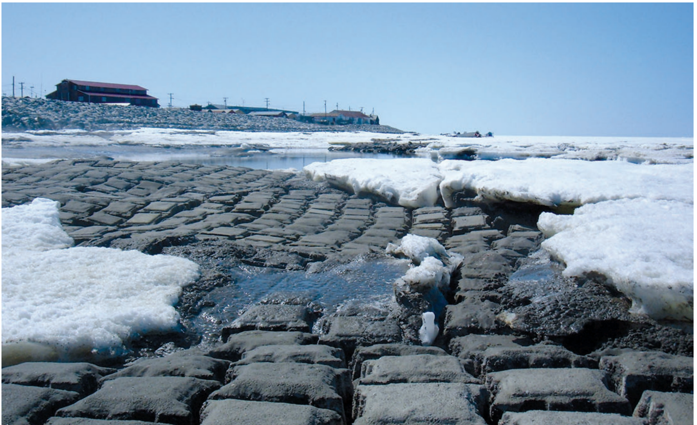
Figure 3: Melting Sea Ice Reveals Prior Control Efforts and the Advance of Erosion toward the Seawall Being Constructed in the Village of Shishmaref, Alaska, June 2008
