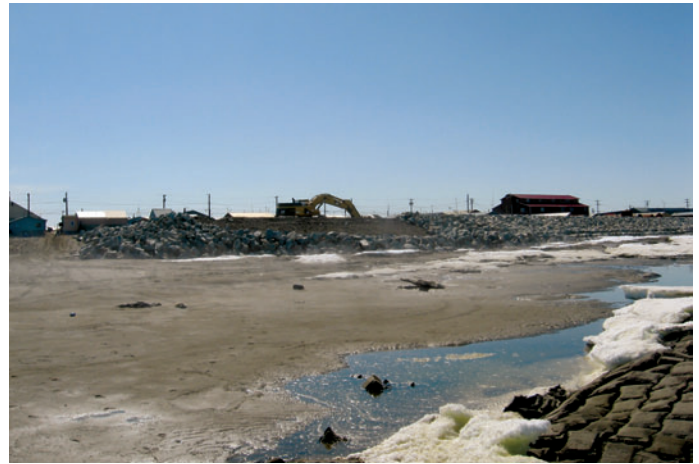
Source: GAO. Shishmaref seawall construction
