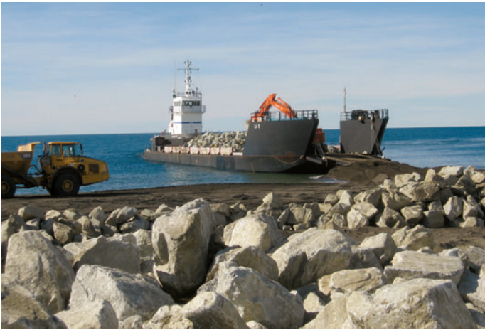
Source: GAO. Unloading rocks for Kivalina's seawall
