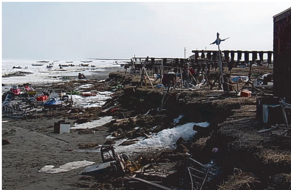
Figure 2: Sea Erosion at Shishmaref (June 2003)
