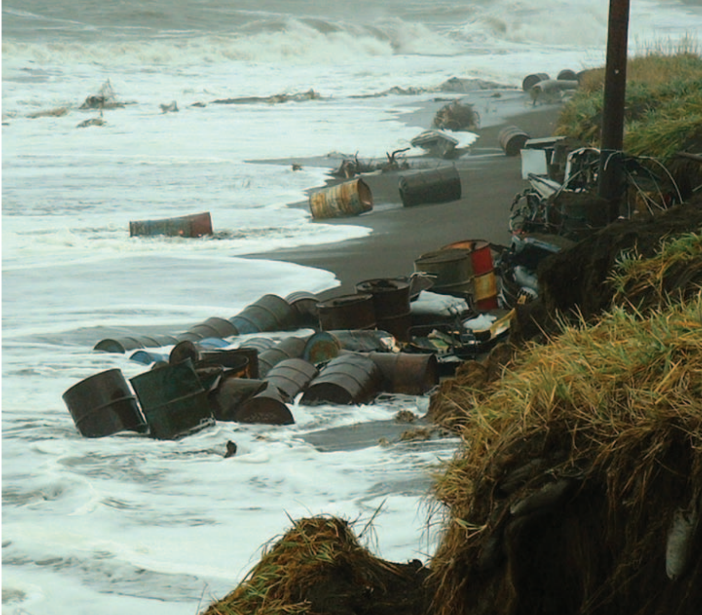
A failed erosion prevention effort. Courtesy of Millie Hawley.
