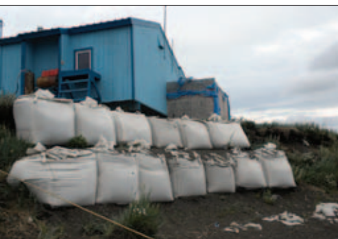
A home on the edge of eroded bank. Michael Brubaker 2010.
