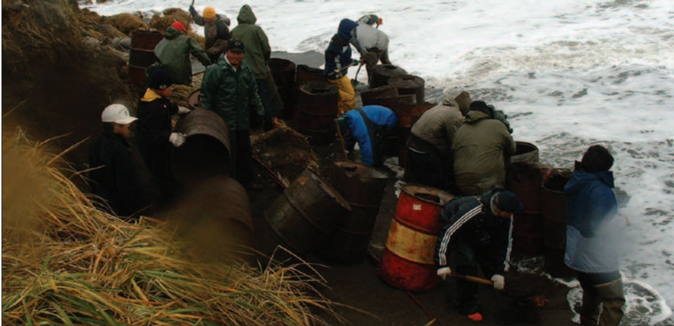
Emergency erosion control. Courtesy of Millie Hawley.
