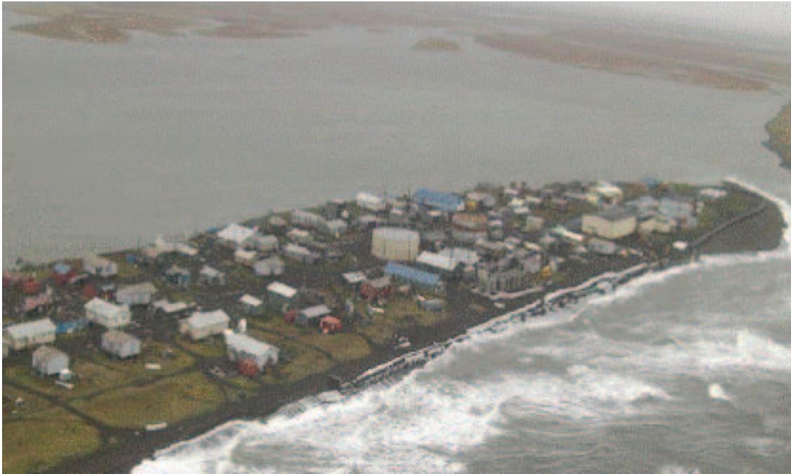
Storm waves threaten Kivalina. Courtesy of the Alaska Department of Transportation.
