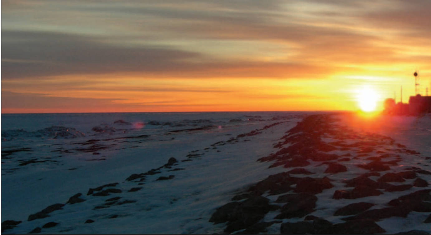
Sunset over the beach revetment wall.
