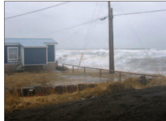
High water in October of 2004. Courtesy of City of Kivalina.
