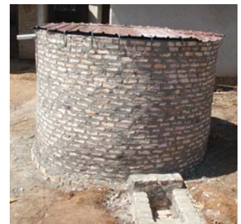
Building a brick-and-mortar water tank (left to right): UMN student Danielle Chase and community member Yasin cover the foundation with banana leaves while it cures, the tank under construction, and the finished tank with cover installed.
