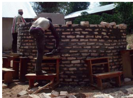
Building a brick-and-mortar water tank (left to right): UMN student Danielle Chase and community member Yasin cover the foundation with banana leaves while it cures, the tank under construction, and the finished tank with cover installed.
