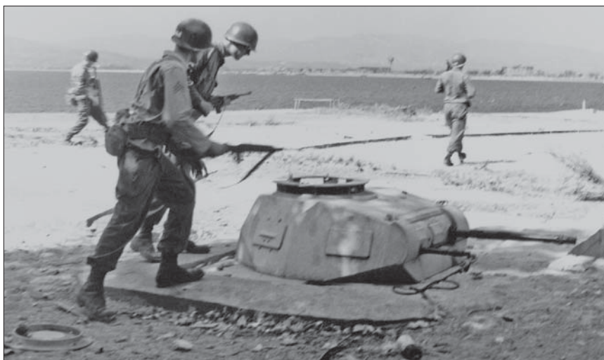
Advancing troops step over an improvised pillbox which has been fitted with a tank turret as armament.
