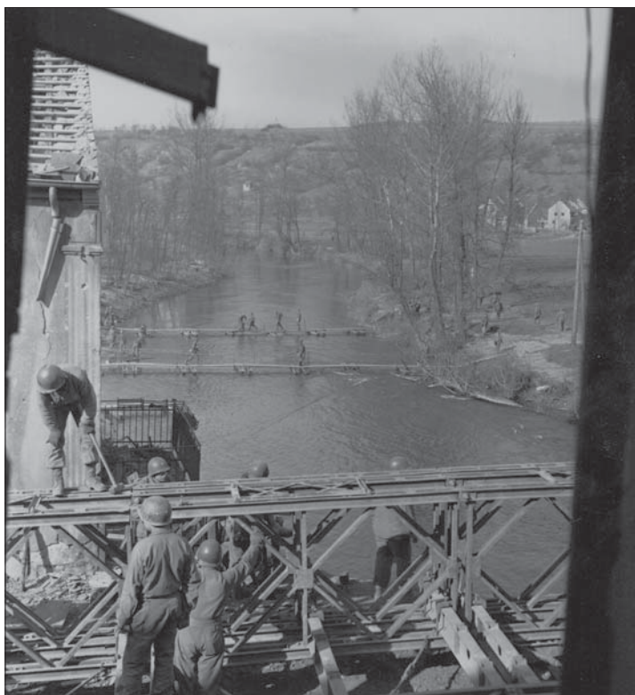
Engineers construct a Bailey bridge while troops cross on a footbridge already established.
