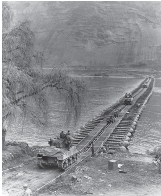
A treadway pontoon bridge is used to cross the formidable Rhine River.
