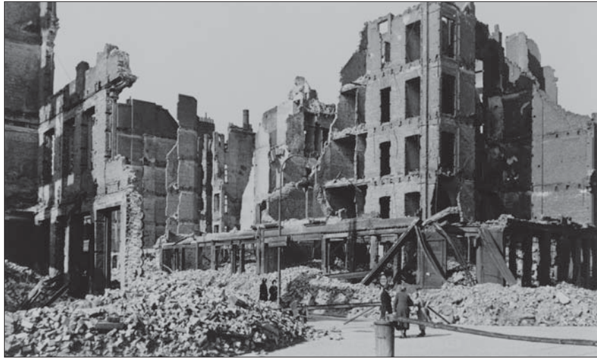
The skeletons of buildings left in Hamburg.
