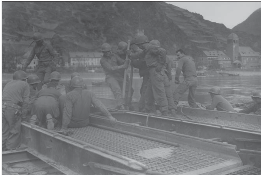
Engineers work hard to quickly build bridges for the allied armies to cross the Rhine.
