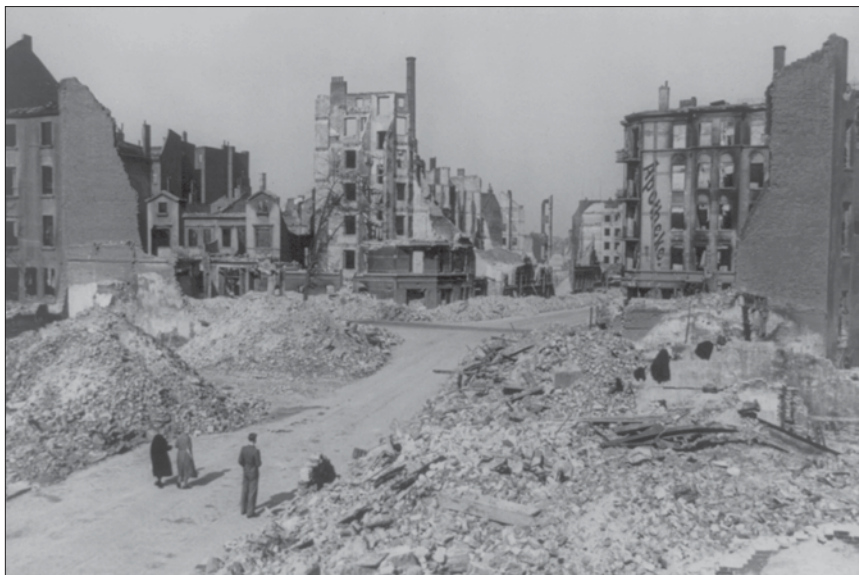
Civilians gaze upon the destruction of Lindernallee, Hamburg, from the firestorm bombing campaign.
