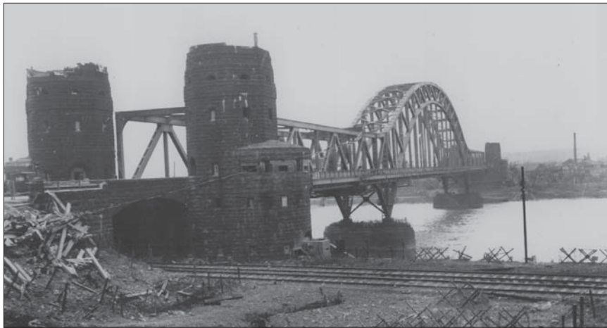
Remagen Bridge prior to its collapse.
