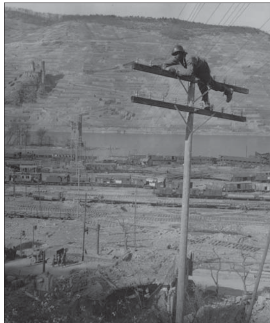
A Signal Corps lineman strings telephone wire in the Rhineland.
