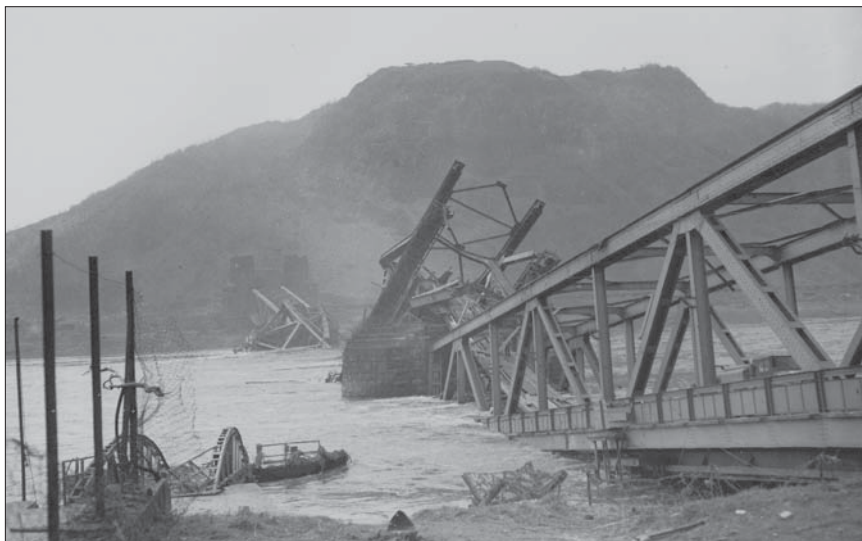
Remagen bridge after its collapse.
