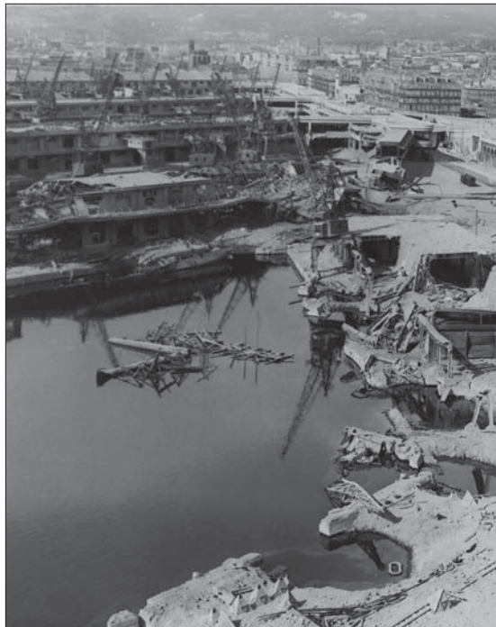
The docks at Marseille after the German attempt to destroy them with explosives before surrendering the city.
