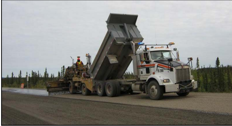
Figure 14: Placing the light-coloured BST.
