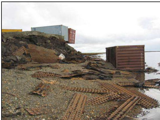
Typical Newtok Erosion
