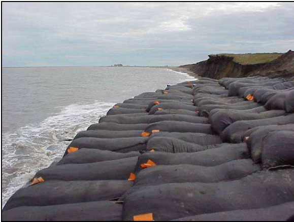
Corps Gravel Bag Revetment in 1999
