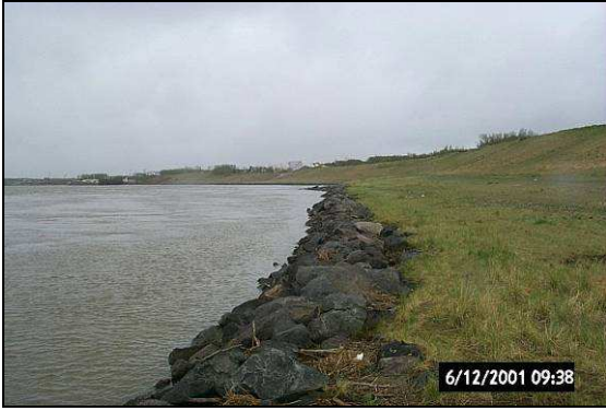
Riverbank Protection at Bethel
