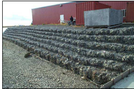
Typical rock filled gabion bank protection
