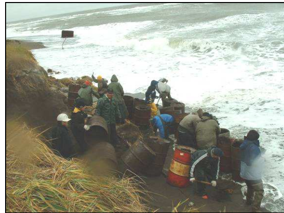
Emergency shoreline protection - 2005
