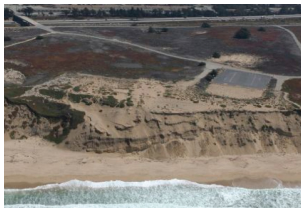
E 4. Once the building and revetment were removed, the beach recovered. 34
