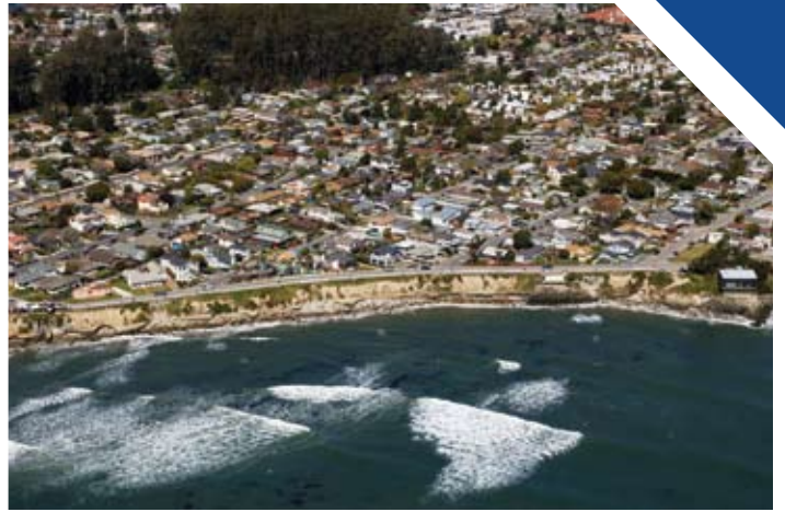
Pleasure Point Seawall - December 2007
