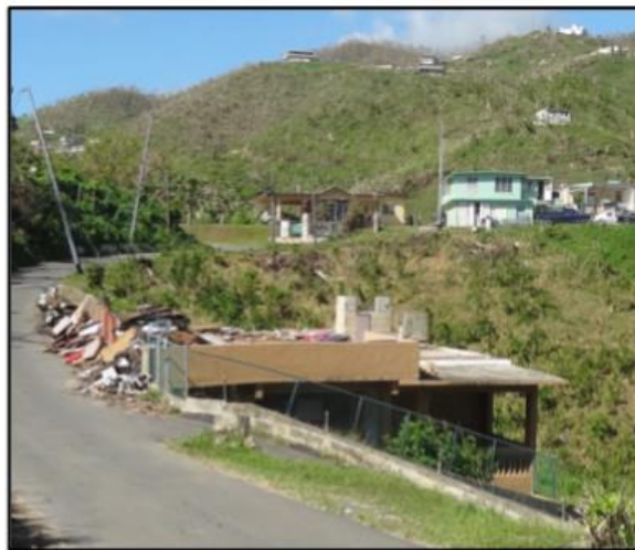
Figure 1. Damage associated with topographic wind speed up
