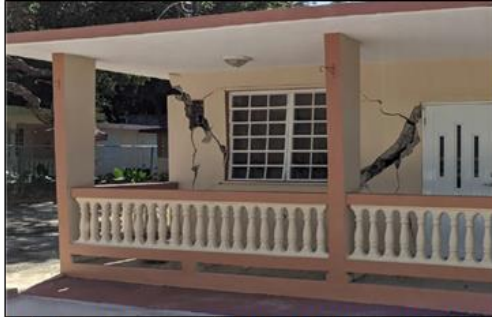
1 Story House: CMU Walls with Flat Concrete Roof
