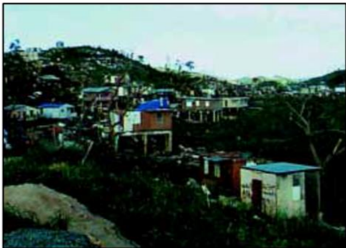
Figure 1. Damage associated with topographic wind speed up
