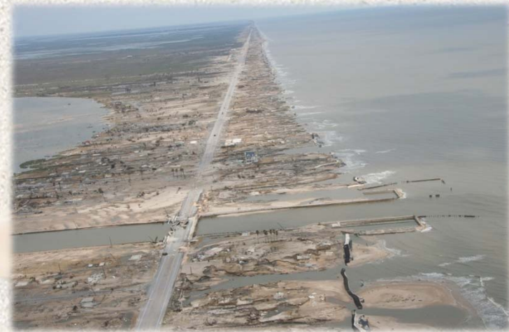
Enhanced building codes allowed one house to remain standing on Bolivar Peninsula, TX after Hurricane Ike. Photo Credit: NOAA
