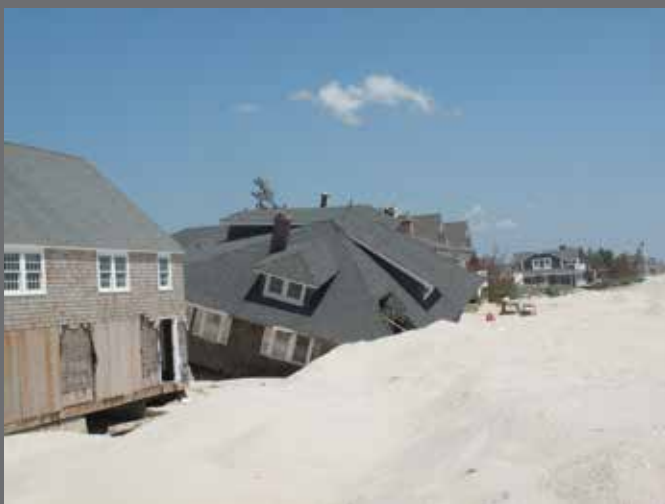
Beach houses in New Jersey were destroyed by Hurricane Sandy. Credit: New Jersey Sea Grant
