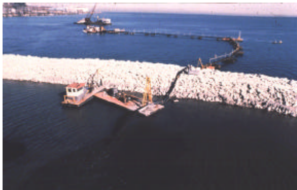
Figure 9. Hydraulic dredge discharge to Chicago Area CDF
