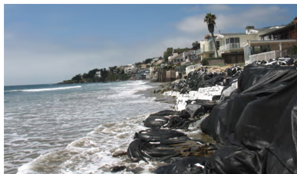
FIGURE 5. Under winter beach conditions, these temporary protection structures in Malibu significantly reduced lateral and vertical access.
