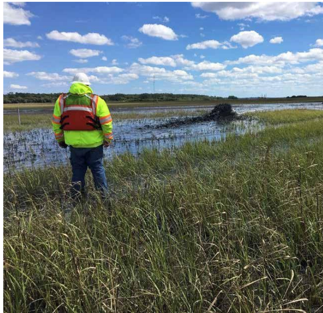
Dredging project manager monitoring dredged sediment placement at the Jekyll Creek Marsh Restoration and Wetland Habitat development Beneficial Use of Dredged Material project, Georgia. (Photo by Clay McCoy, USACE Jacksonville)
