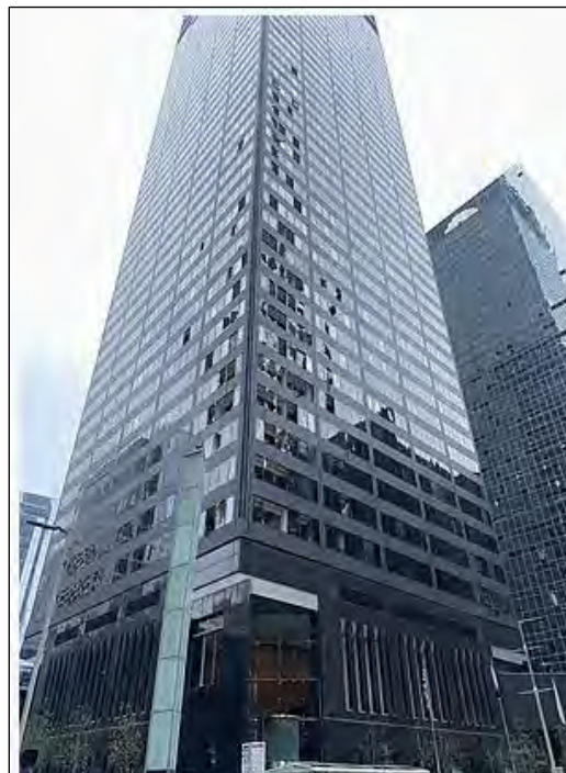
Picture 5: Windows blown out of CenterPoint Energy Plaza
