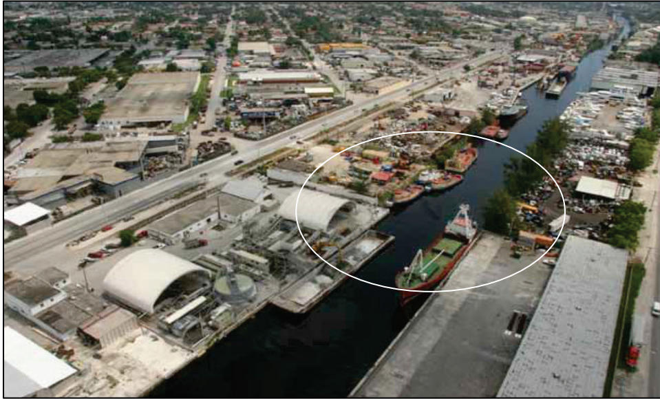
Figure D-2. Photograph of Boskalis-Dolman physical separation system, Miami River, Florida (courtesy Bastiaan Lammers, Boskalis Dolman).
