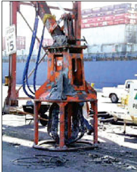
Figure D-10. Mixer for in-barge mixing of amendments for sediment S/S.
