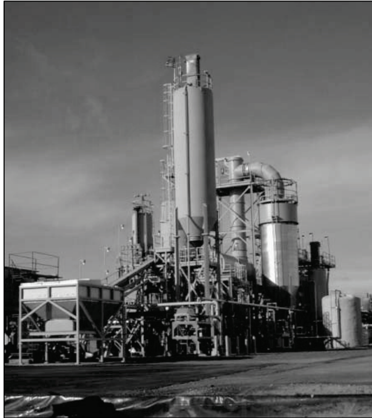
Figure D-13. Cement-Lock® demo plant (Mensinger 2008).
