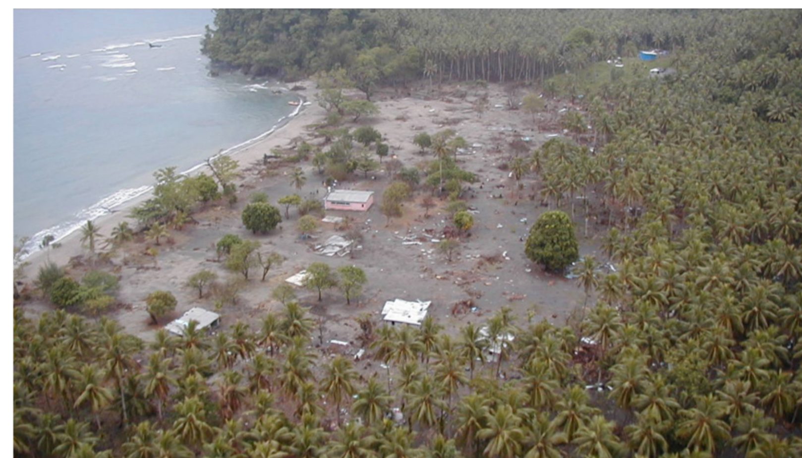
The village of Baie Martelli, Vanuatu, was destroyed after the 1999 tsunami. The large concrete village church (center image) was one of the few structures that remained standing following the tsunami. However, water surged over the top of the church (over 4 m above ground surface), crushing its corrugated metal roof. (Image Credits: Costas Synolakis (left), Utku Kanoglu (center, right))
