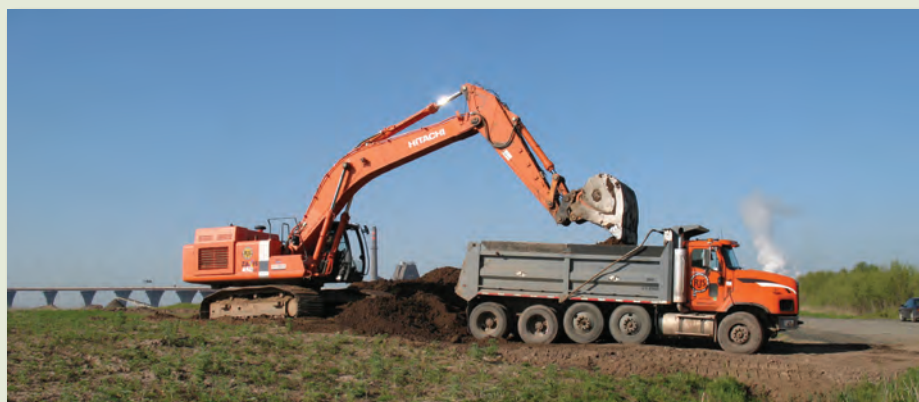
Removing dredge material from Erie Pier in Duluth.
