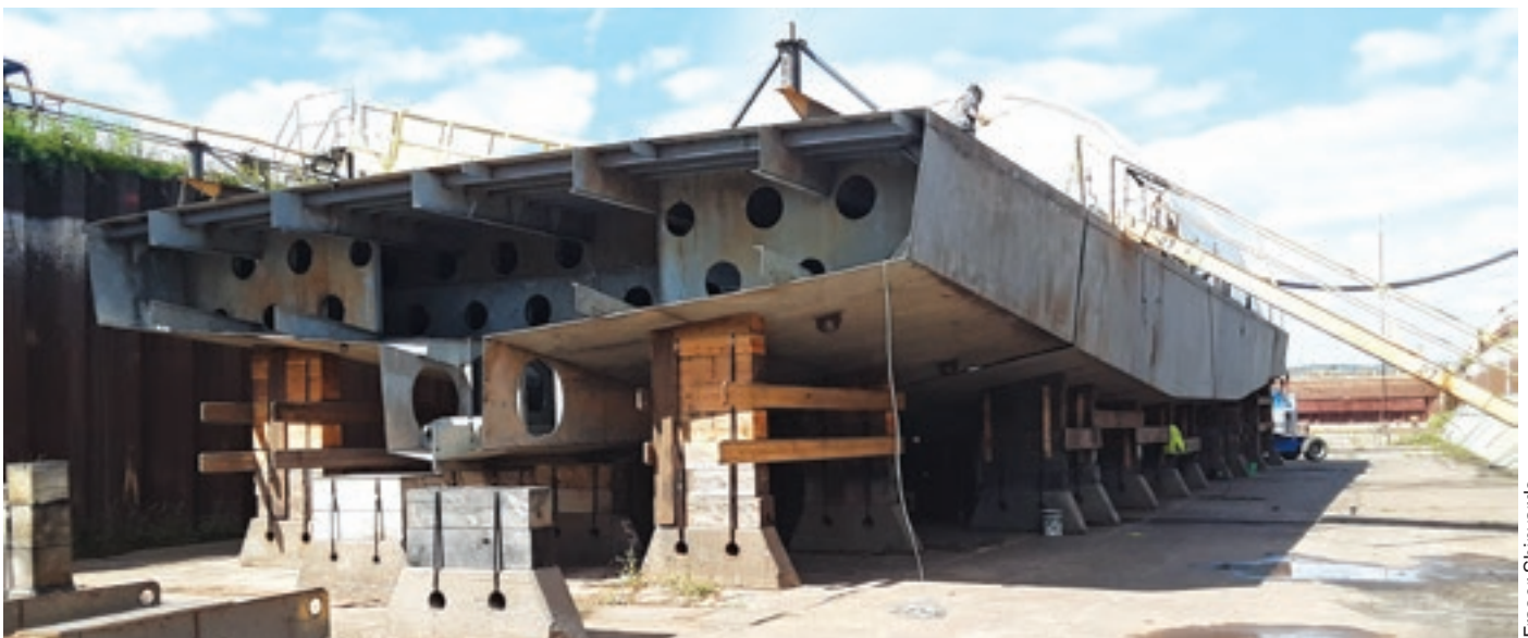
The hull of the Mary Ann Market rests at Fraser Shipyards awaiting the final hull section/module. When fully completed, she’ll sail to her new home port of Put-in-Bay, Ohio.
