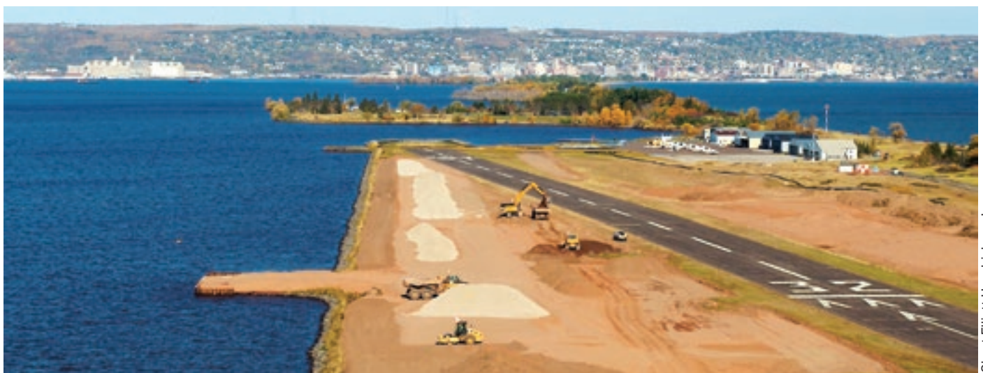
Heavy equipment smooths the way for runway relocation at Duluth’s Sky Harbor Airport. The project entered its final phase earlier this fall.
