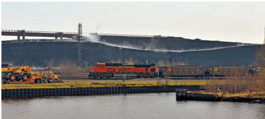
Midwest Energy's coal-handling system is a model of efficiency. Here a 123-car unit train arrives with coal from the Powder River Basin. Two trains' full of coal will fill a Canadian laker for shipment to Quebec.
