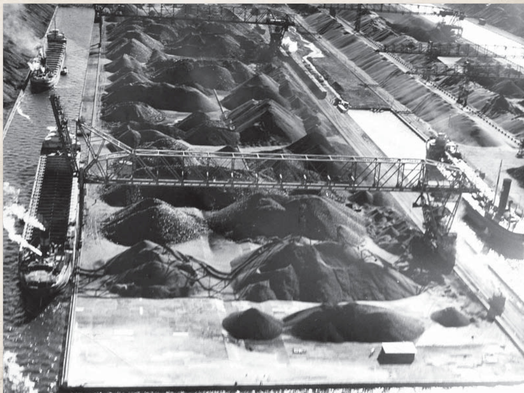
The trestle, or moving bridge, was a key component in handling cargo at the early-20th century coal dock.
