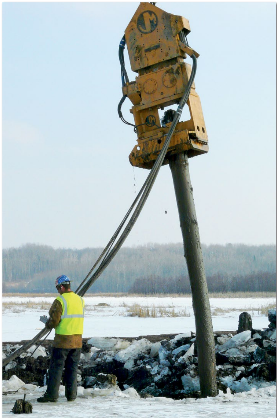
Pulling a piling from the bottom of Radio Tower Bay.
