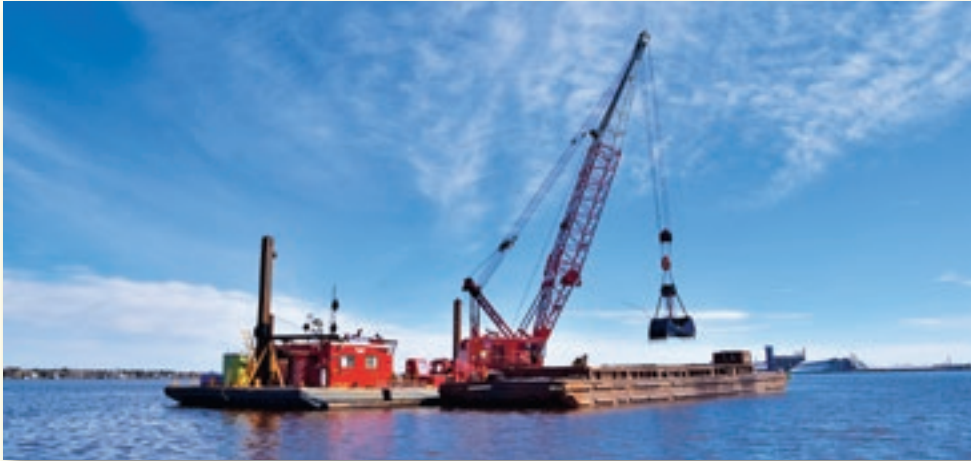
Marine Tech crews dredged the East Gate Basin in 2017.
