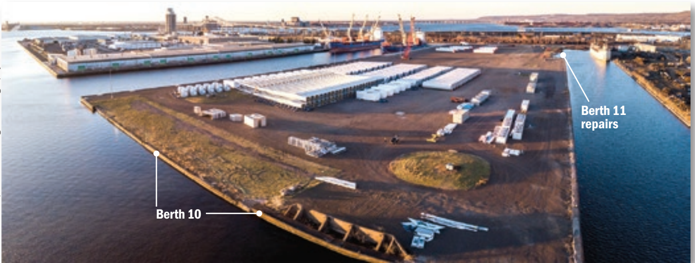
Repairs to Berths 10 and 11 are on the docket for the 26-acre Clure Terminal Expansion.
