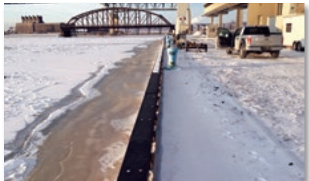
New fenders are in place for the 2018 season.
