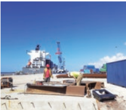
NORDIC crews perform emergency repairs at Port Lafito.
