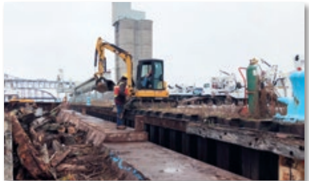
Old fenders on Berths 5-7 are removed.
