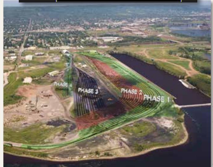
Site drawing for the new Hallett Railroad Storage and Services company, located on Hallett Dock No. 6 in Duluth.
