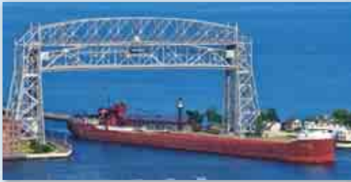
The Hon. James L. Oberstar clears Duluth's Aerial Lift Bridge on Aug. 31.
