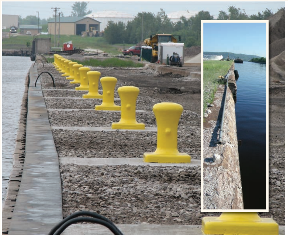
Once-crumbling dock walls at Hallett Dock No. 8 (inset) are being rehabilitated in a $3 million project.
