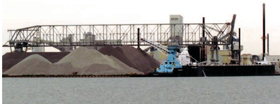
Graymont's 640-foot man-trolley has become a fixture at the plant in its century of service. Here, the tug-barge Ken Boothe Sr./Lakes Contender discharges limestone.
