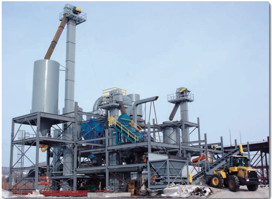
Who needs an exterior? Duluth Minerals got its processing equipment in place — and went to work uncovered. Operations now. 'Skin' later this year.
